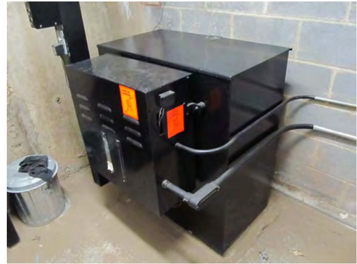
Typical hydro-mechanical and controller/dispatcher equipment for each of the building's two elevators
