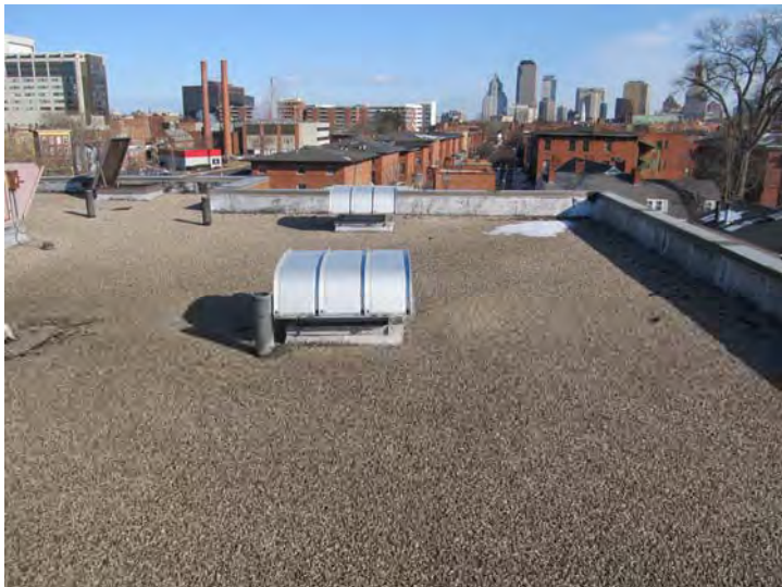
Original built-up roof covering typical on all portions of building
