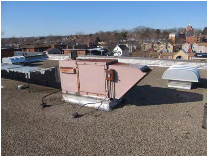
Rooftop-mounted make-up air unit located at four-story section of building
