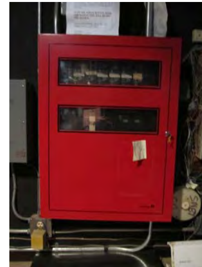
Original zone-type fire alarm control panel is serviceable but at or near the end of its expected useful life
