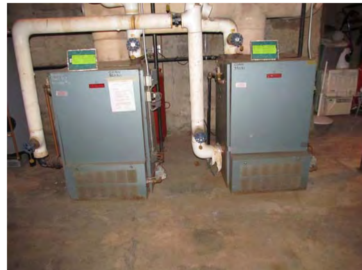
Original cast iron boilers for production of hydronic heat
