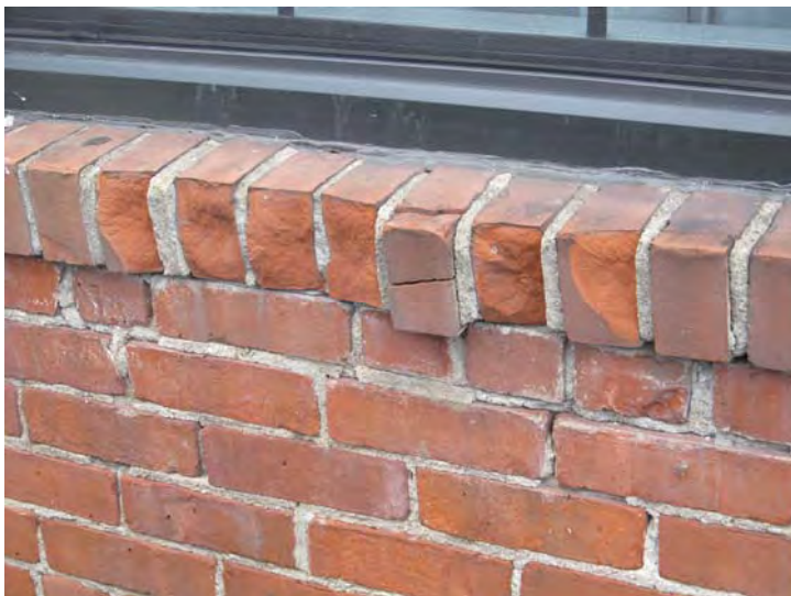
Isolated areas of brick spalling also noted
