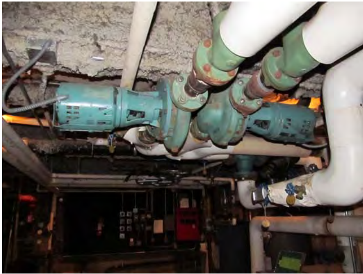
Inline circulating pumps for distribution of hydronic heat throughout the building
