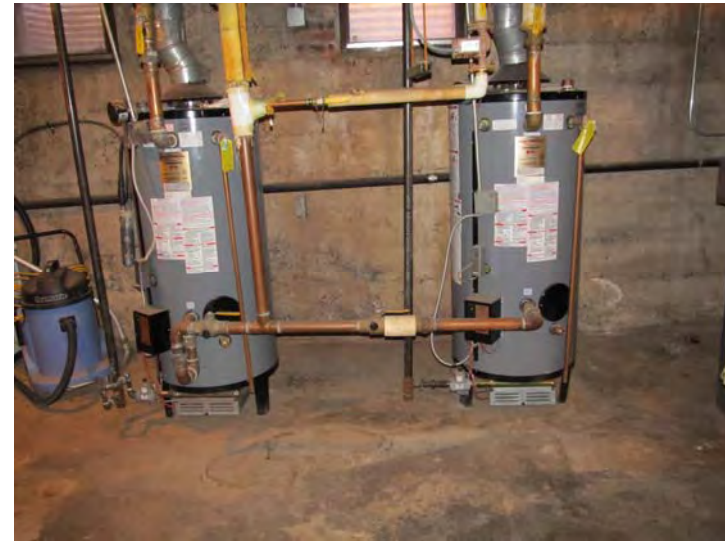
Two freestanding tanks produce domestic hot water for the entire building
