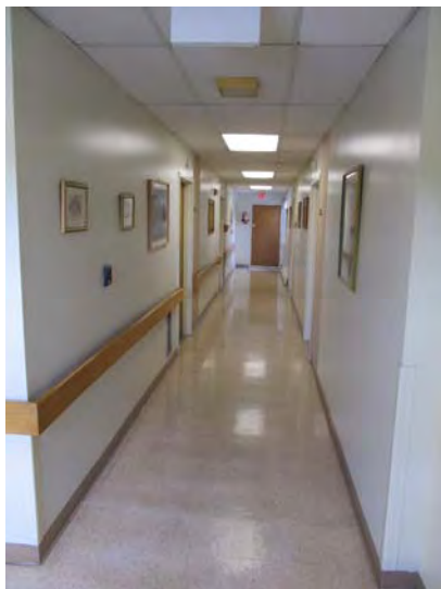
Common halls at upper floor levels have original vinyl tile floor coverings
