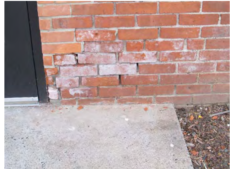
Isolated areas of mortar loss noted around building
